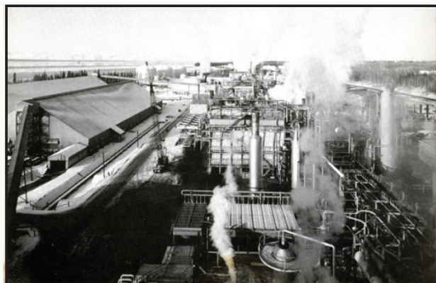
Natural gas, atmospheric nitrogen and electricity are utilized to produce 1,500 tons per day of NH 3 at a West Coast manufacturing plant.
